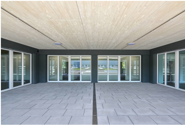
Entrance area with wooden ceiling
