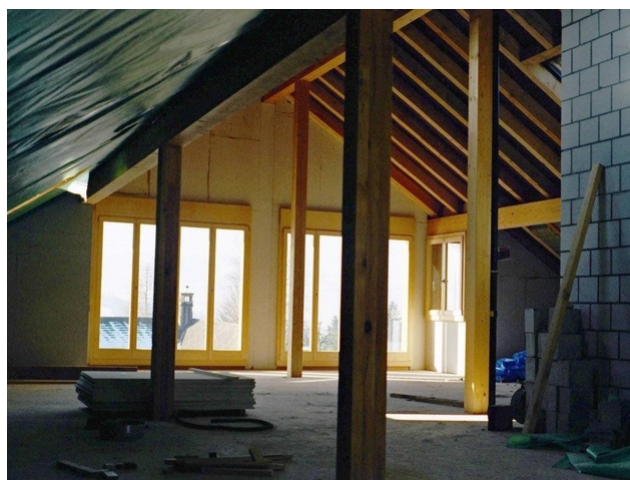
In the attic
