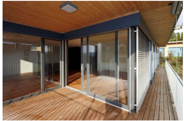
Exterior view south apartments
