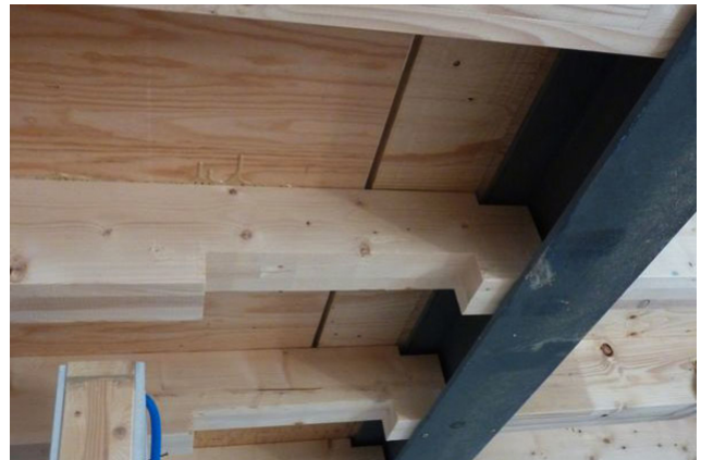
Cutouts for building services installations in the rib elements of the floor slabs
