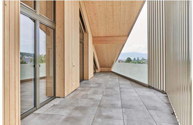
In the village center of Gretzenbach in the canton of Solothurn, a timber building with twelve apartments and a village store was built. The balconies cantilever over 3.5 meters - without any disruptive supports. An ingenious, suspended construction makes this possible.
