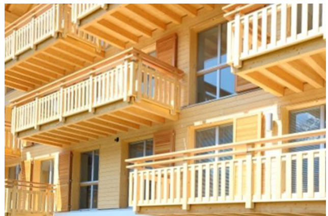
Facade with balconies, photo Wenger Windows Wimmis
