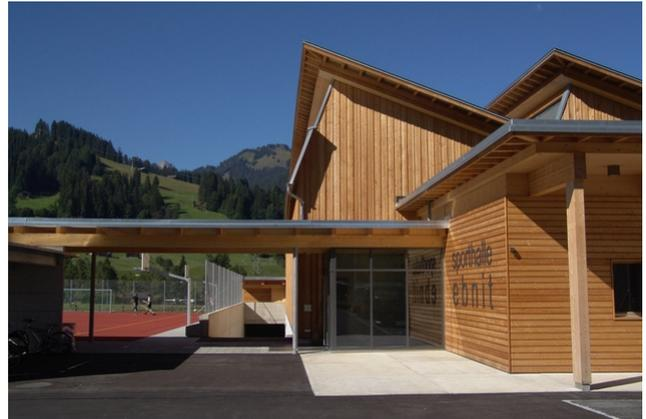
The executed project, a 3-fold gymnasium with combined steel-wood trusses, emerged from an architectural competition in 2002. With the orientation of the shed roof to the south, it is possible to directly use solar energy passively.
