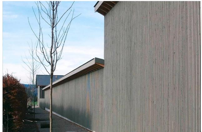
The Polo Park Zurich has relied entirely on wood as a building material for its new center. Both the operations building and the various stable buildings with the horse stalls have been realized as timber frame buildings.
