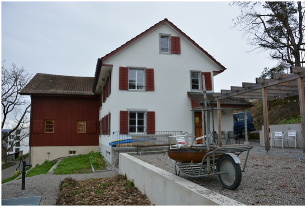
Exterior view QuarTierhof
