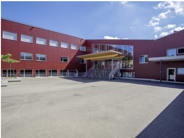
One unit: on the left you can see the gymnasium, next to it the connecting wing, on the right the renovated school building
