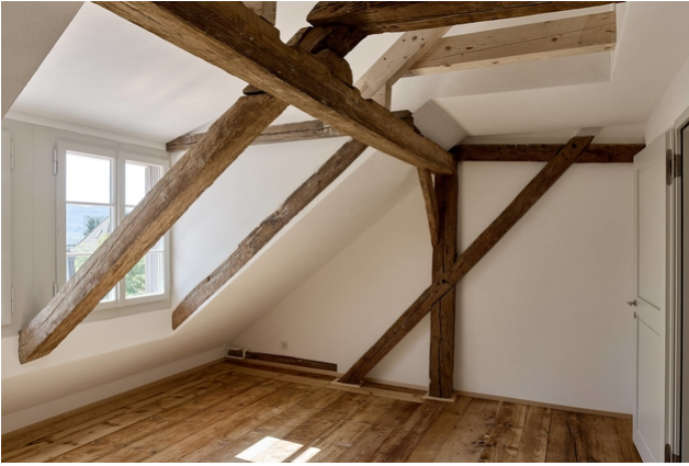
Existing roof truss
