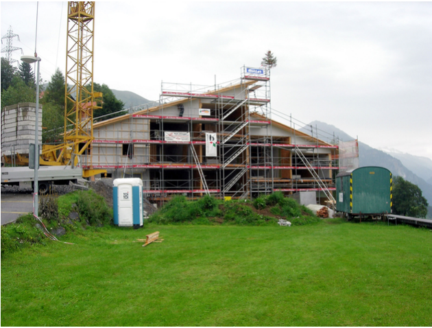
Shell of the building
