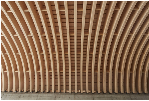
The wooden structure remains visible from below
