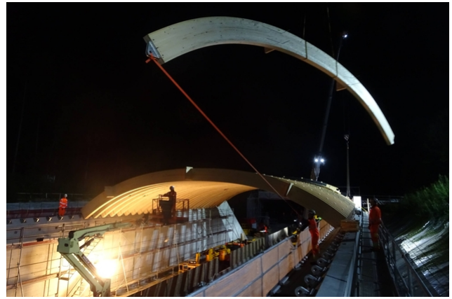
Assembly work at night
