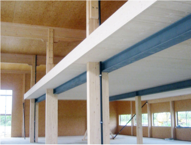
Gallery with 1t payload per m2
