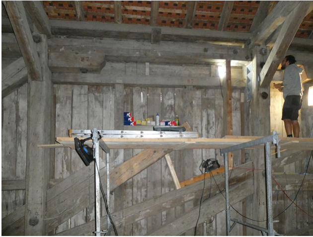
Strut renovation of the bridge
